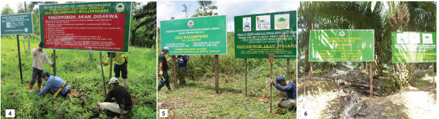
(4) Fixing warning signboards and (5)&(6) Fixing forest reserve signages.
